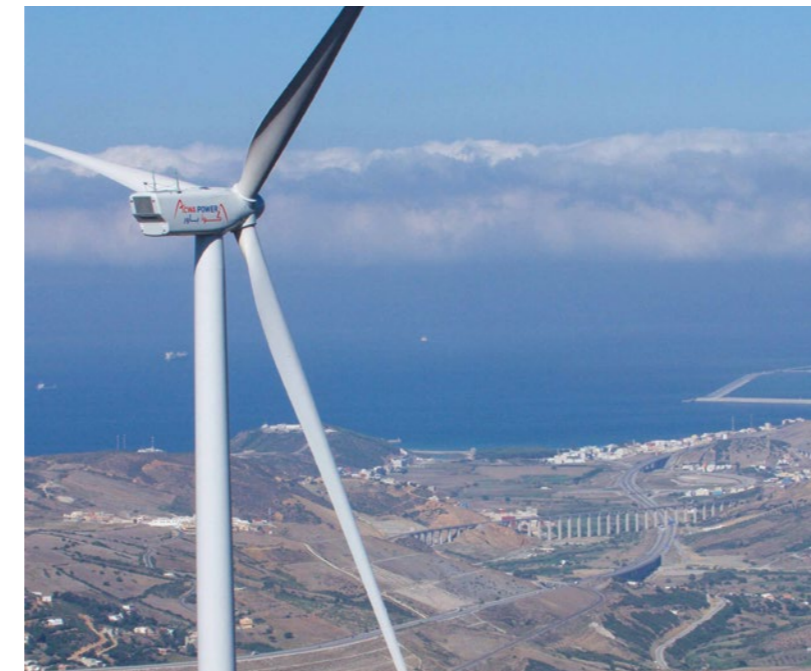
Wind energy in Tangier-Tetouan, Morocco
